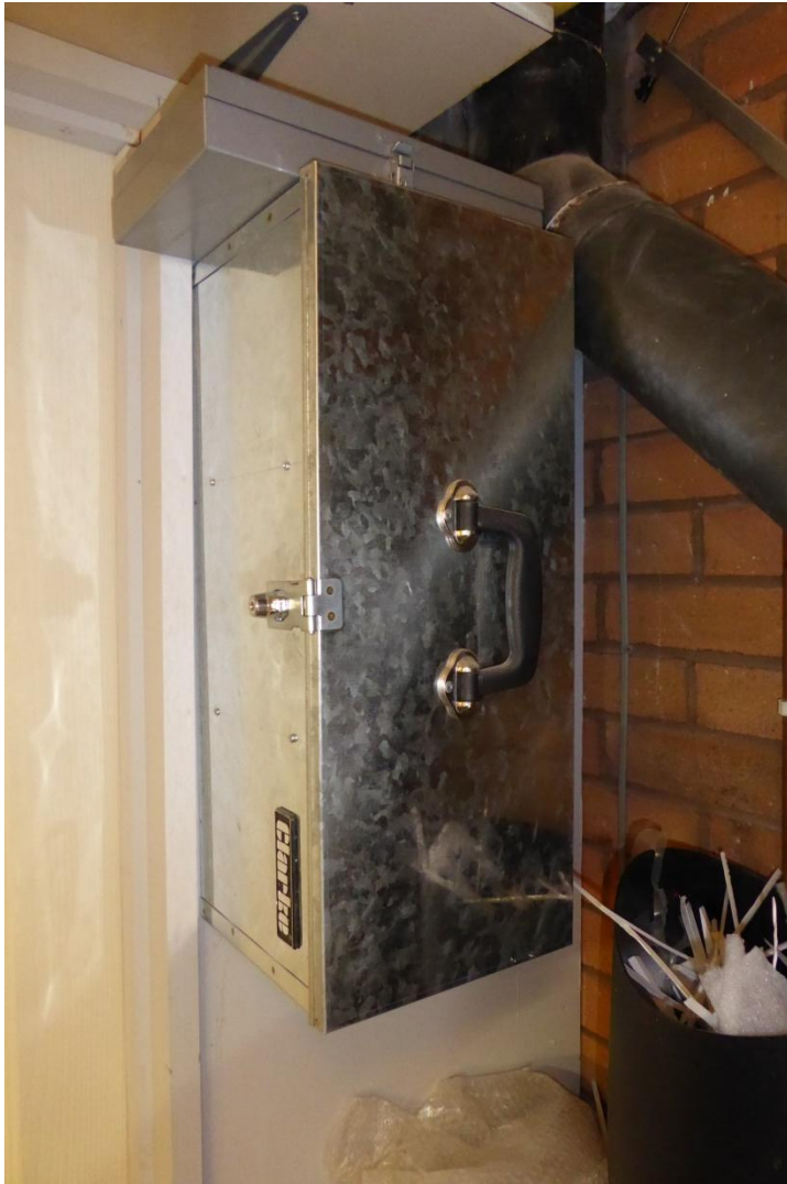
Small box on top (small batteries)
